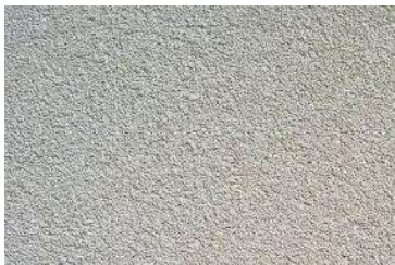
CSR Hebel Power Wall system with acrylic render textured finish.
