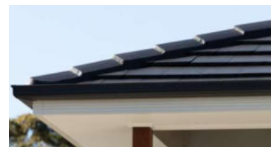
Standard ridges to all tiled roofing
